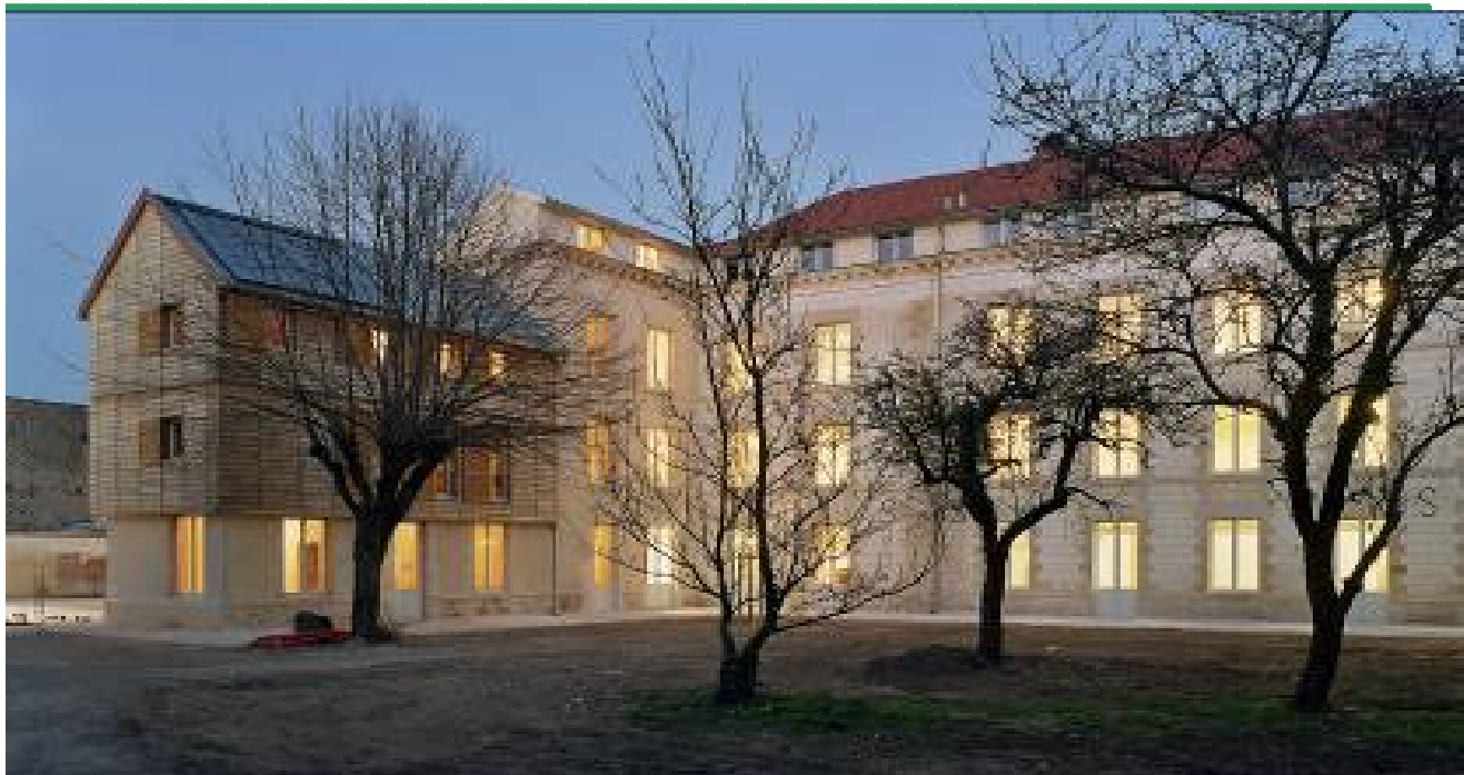
Figure 13 Stone building renovated with hemp-lime plaster
