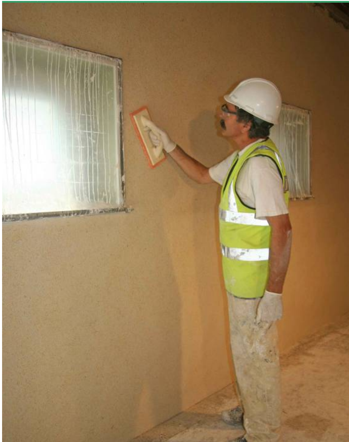
Figure 12 Applying hemp-lime plaster
